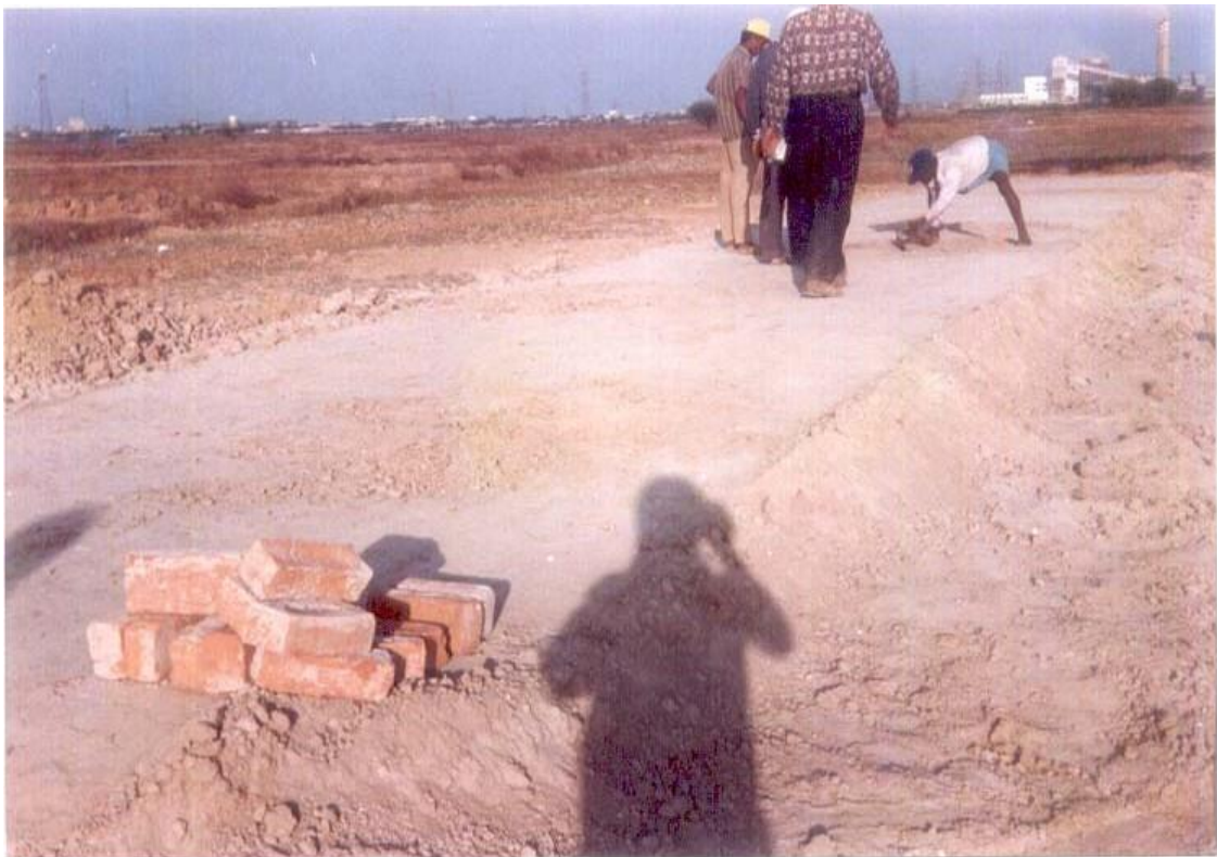
FIG.4 – VIEW OF COMPACTED SURFACE (SOIL WITH 20% FA)
